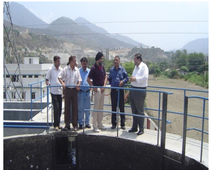
Picture 15: STP at Sringar
