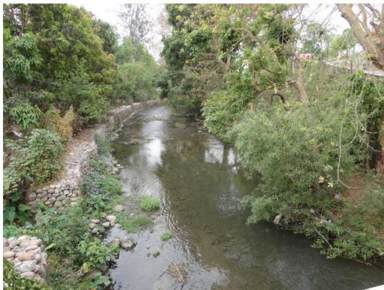
Picture 23: Image of Rambha river at Rishikesh (Uttarakhand)
